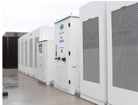
McCrary Battery Storage Demonstration
