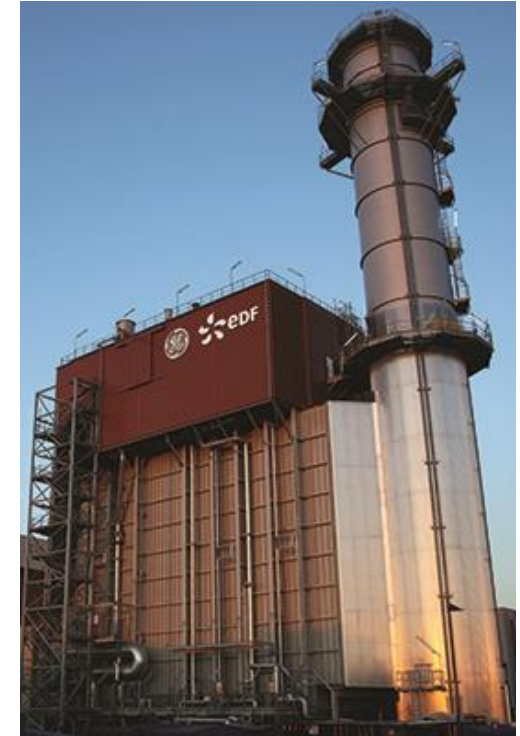
Backup Boiler for Depleted Storage
